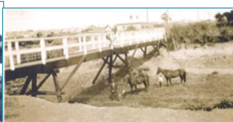
Dawson St Bridge over Moonee Ponds Creek 1926
