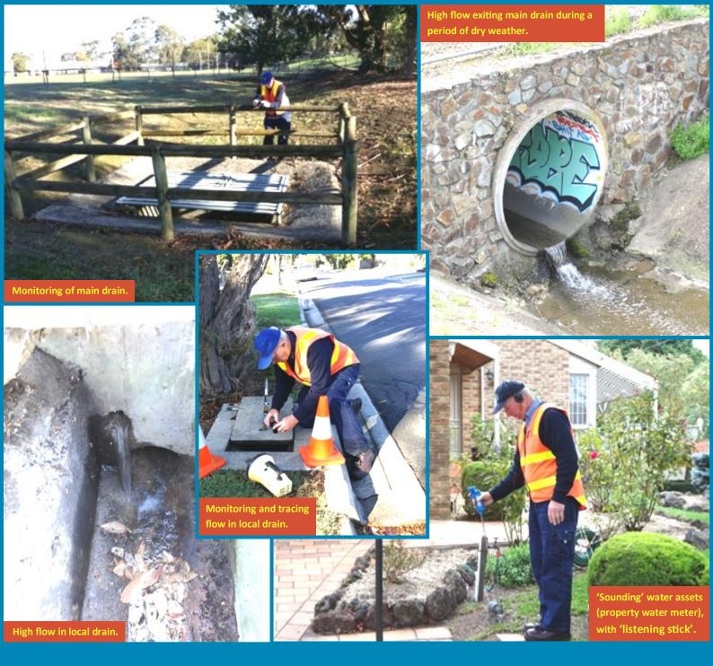
"Many of the monitoring points are located at the outlets of main or large stormwater drains managed by either the local council or Melbourne Water. The drains exit into the streams, creeks and rivers. If an unusually high flow is observed at the monitoring point, particularly in periods of dry weather, the flow is traced upstream via inspection manholes in the drainage system. The 'chaser' is armed with detailed plans of the water and drainage systems for each location.
