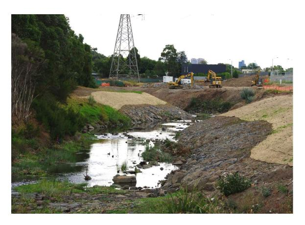
Figure 134. Erosion control works along a section of Gardiners Creek, 2014. Source: Author image (2014).
