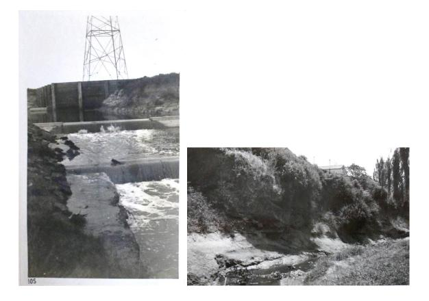
Figure 50. A section of Gardiners Creek, c.a. 1940s, with weirs, and timber retaining wall to control erosion. Moonee Ponds Creek bank erosion in 1955. Source: PROV, VPRS 8609/P32, Unit 7, PA17
