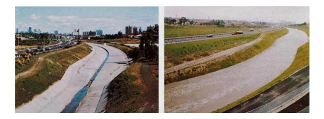
Figure 94. The longest section of realigned creek course during normal and flood flows. The freeway is along the original creek bed. Source: MMBW (1976).
