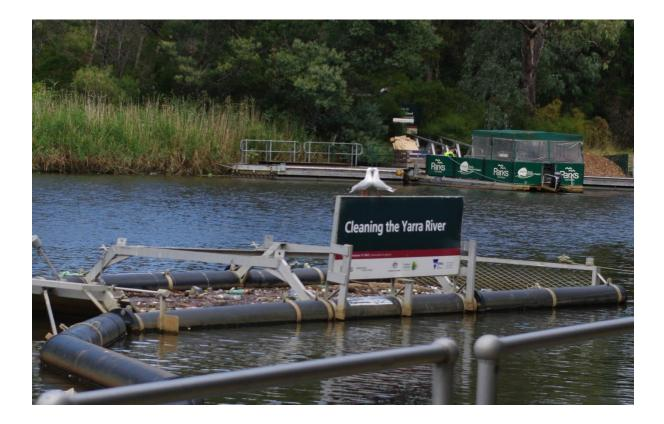
Figure 144. Litter trap on the Yarra near a main drain outlet. Source: Author photo (2016).
