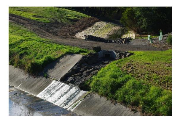
Figure 139. Restoration of the last 100 metres of a previously undergrounded, un-named tributary of the Moonee Ponds Creek. Engineered for stormwater drainage using designed wetland system with indigenous vegetation to filter the water and create habitat. Source: Author image (2017).
