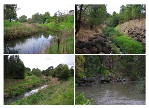
*Figure 55. Examples of earthen trapezoid channels designed by the MMBW. From top left, Merri Creek; Ruffy Creek; Darebin Creek, and bottom right, Koonung Creek. Source: Author photos (2017)*
