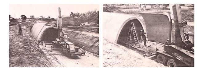
Figure 117. Undergrounding the lower section of the Koonung. Source: PROV, VPRS 8609/P0021, Unit 477
