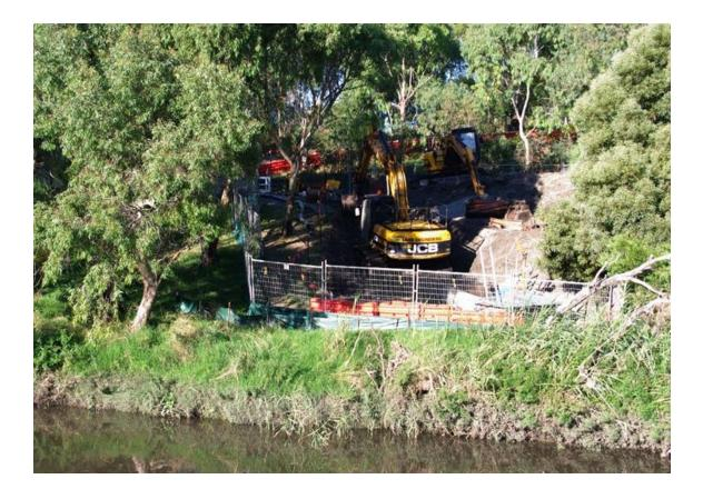
Figure 70. Rehabilitation work on a main trunk sewer along the Merri Creek. Source: Author photo (2017).
