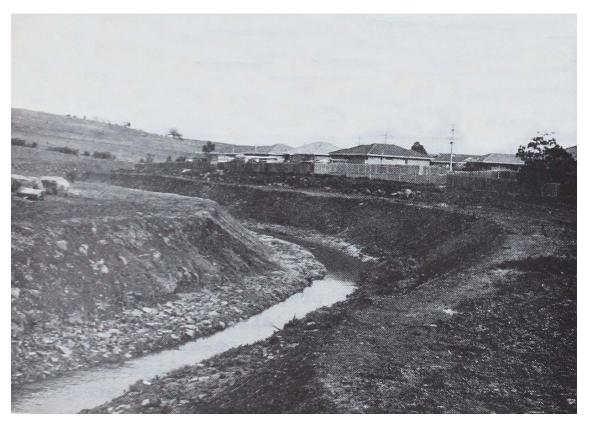
Figure 137. The same section of creek following modification for flood mitigation and control. Source: PROV, VPRS 8609/P0021, Unit 477
