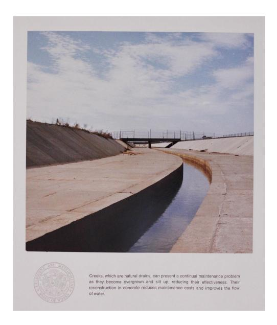
Figure 121. MMBW drainage division, 1973, image of canalised creek including description of creeks as 'natural drains'. Source: PROV, VPRS 8609/P21, Unit 110
