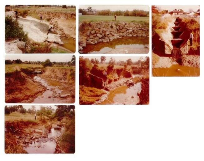
Figure 115. Damage to erosion control structures along the Koonung. Source: MMBW (1979).
