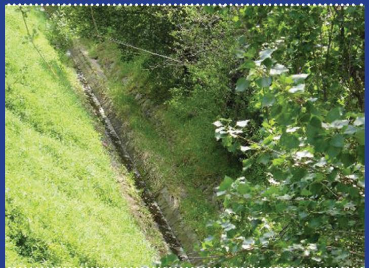
The section that still flows above ground today north of Glenbervie Station is a remnant of this era. This section is two bluestone pitches wide, with sloping sides two bluestone pitches high and retaining walls set back on each side. It has been deemed significant by the Heritage Council of Victoria for “showing how the natural environment was modified in the interwar period...to reduce the effects of flooding...due to increased run-off from urban development”. (Heritage Vic).
