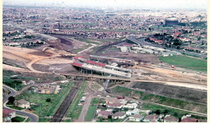
This aerial view from the 1960s, provided by Maurice Austin, shows work in progress on this section of the freeway, with its elevated section at lower right being created from the spoil from the immense new cutting that ran alongside Essendon Airport. The photo also shows Strathmore High School in the background, just after its old creek bed had been filled in.
