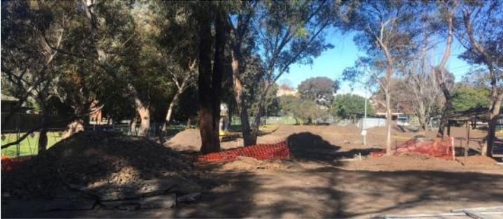
Earth works for the Gavin Park wetland along the Westbreen Creek corridor commenced in July but unfortunately uncovered a significant amount of asbestos. This caused a month-long delay in the program while the site was made safe and an asbestos management plan implemented. Clean up works are nearing completion and it is still anticipated to have the major construction elements completed by December.
