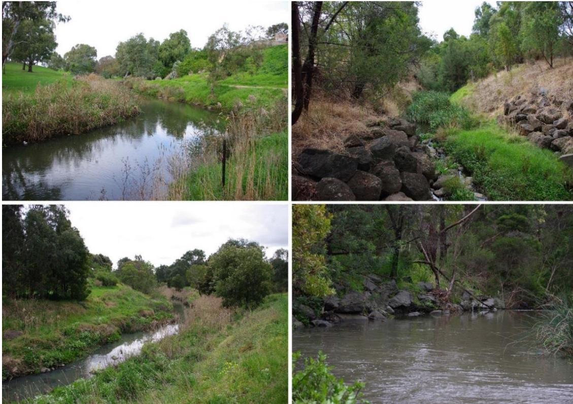
Figure 55. Examples of earthen trapezoid channels designed by the MMBW. From top left, Merri Creek; Ruffy Creek; Darebin Creek, and bottom right, Koonung Creek. Source: Author photos (2017)
